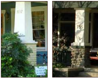
Porch columns of plaster or wood feature a masonry base
