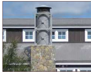
Chimney treated as large vent stack
