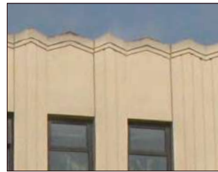
Parapet with serrated coping of plaster
