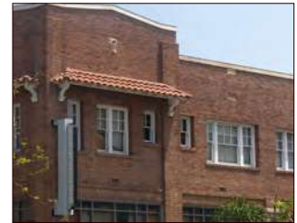
Wall plane with pilasters, lintel expression, and recesses at upper windows
