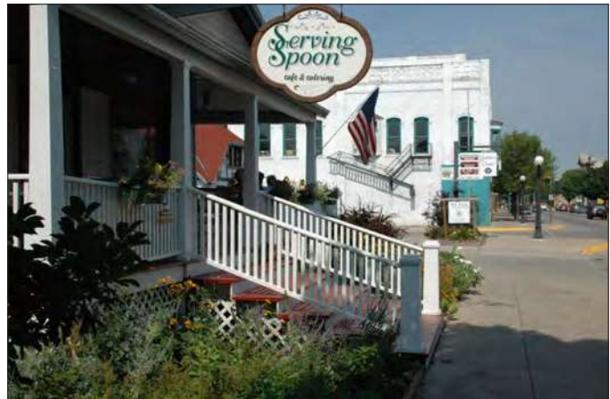
House-form buildings with porch frontages transition from the more intense Downtown Core to the Monterey Street zone.
