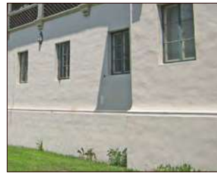
Simple planes, base set off w/ plaster molding at floor level
