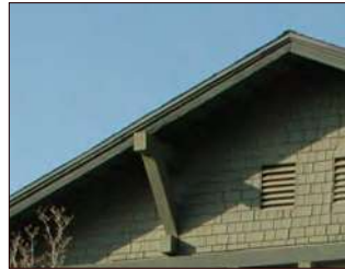
Roof overhang, wooden eave with exposed rafters
