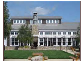
Monitors on roof ridge.
