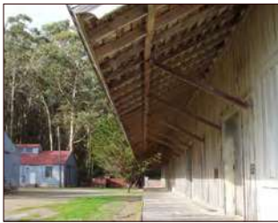
Roof overhang supported by wood struts, decking boards visible
