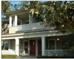
Balcony for upstairs dwellings over full width porch
