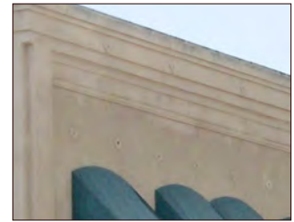
Wall plane, plaster recesses
