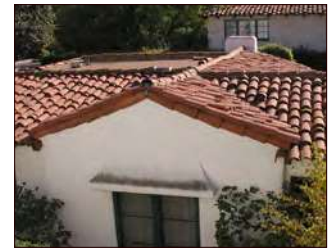
Roof with gable end and flat roof section at rear
