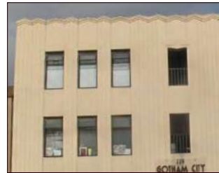
Plaster pilasters and window patterns express underlying structural framework
