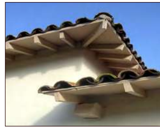
Roof overhang, wooden eave with exposed rafters
