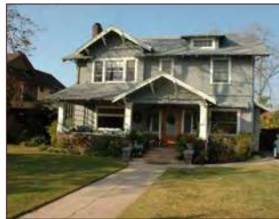
Simple massing, asymmetrical gable, central entry
