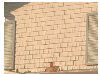
Above and Top: Shingle siding provides texture and interest to the large wall planes
