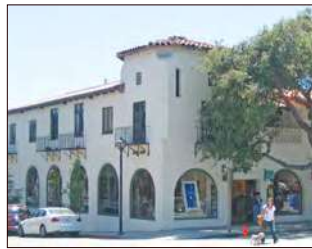
Single volume, corner tower
