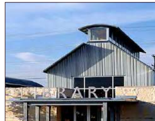
Metal roof, monitor
