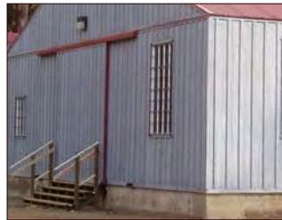
Sliding, oversize door, metal windows
