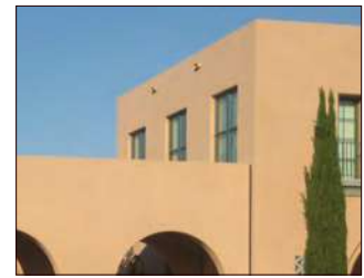
Flat roofs, w/ scuppers
