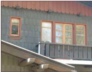
Combined patterns of vertical siding above shingle siding, and vertical balcony planks
