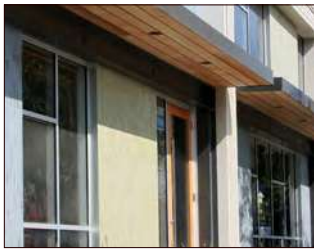
Openings are recessed into facade
